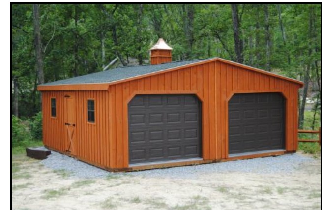
Completed garage in a few hours!
