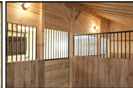
One sliding door and one window per stall; oak kick board 4' high
