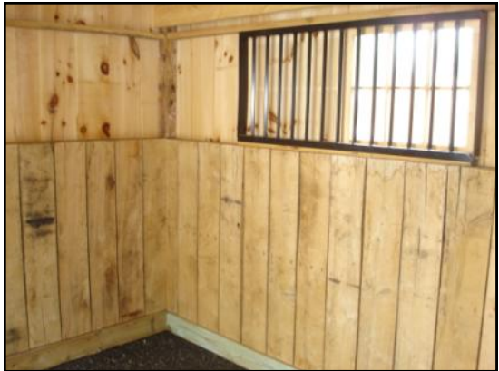
Inside of stall - Kick board and window with metal grill; No floor
