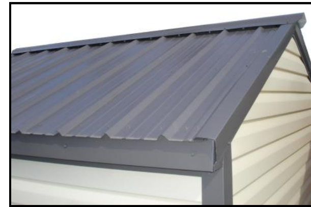
30 Year metal roof (insulated)
